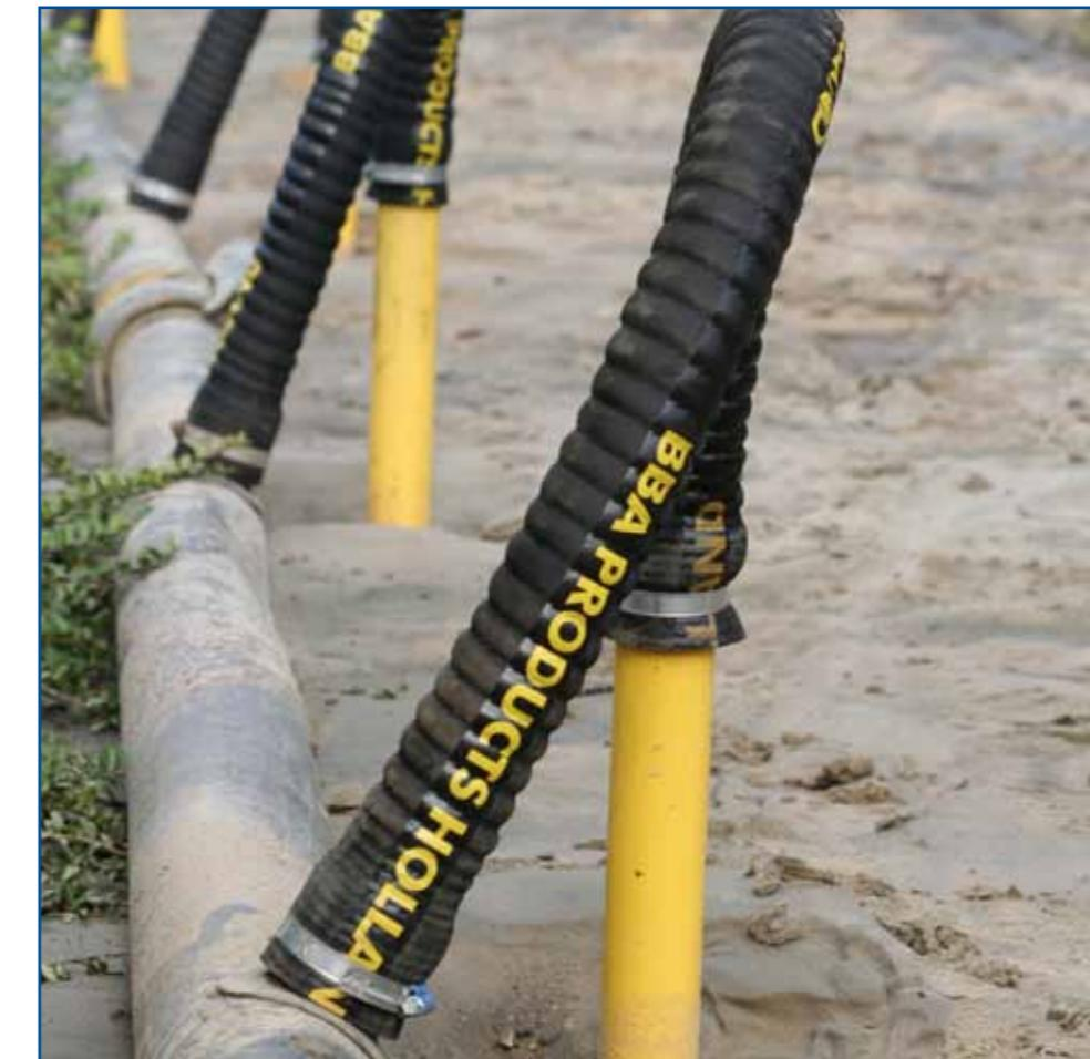
Our application designed wellpoint filters are very light in weight and extremely shock proof. It is a pleasure to use the filters and they are very easy (hand pulled) to remove from the ground and ready for use again.
