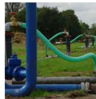
Reducing the groundwater level can have a major impact on the environment or surrounding structures. Groundwater recharge consists of returning the abstracted water to the ground in order to prevent damage, and involves the use of different devices, such as well water filters, well caps and pipes. Leave the selection of the materials to us so you can focus entirely on your drainage project.
